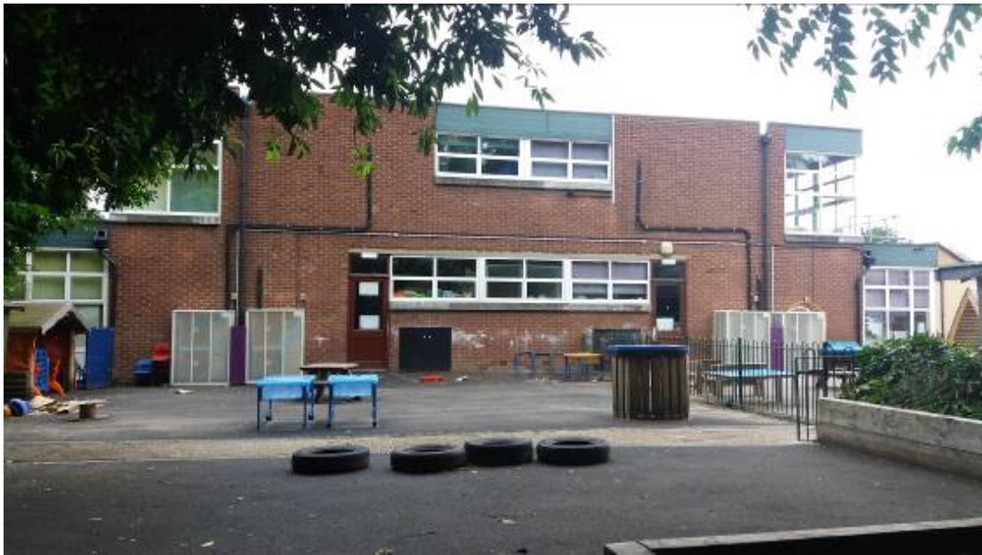
Remaining school building to be demolished
